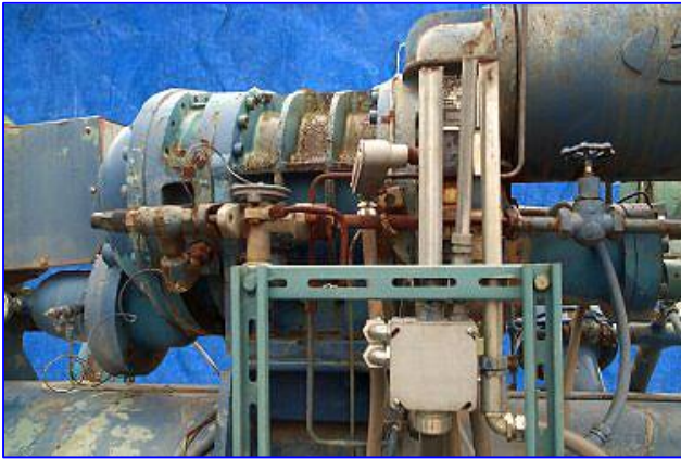
Second Compressor Model: RWB126B, S/N 2512X421, REFRIG NH3, Vol. Ratio-----2.4, Max Speed-----3,600 RPM, Max Pressure--300 PSIG.
