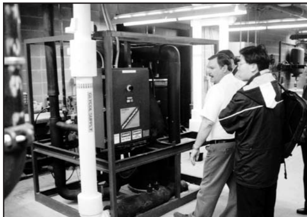
Mr. Rick Book of Mid-American Energy demonstrates the ice slurry system to visitors from China.
