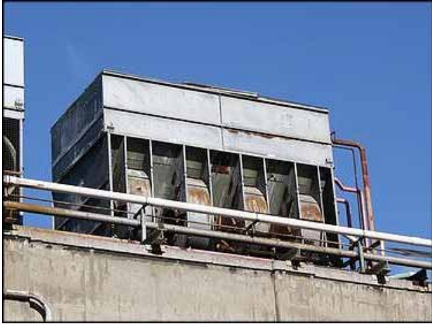
BAC Evaporative Condenser – 400 Ton
