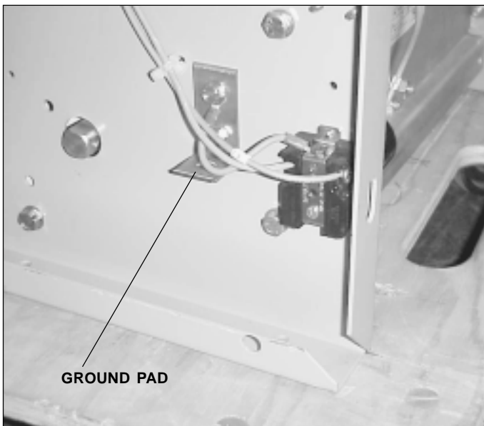
Fig. 15 Contactor Ground Pad
