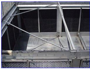
Optional Accessories to include: Stainless Steel Basin, Cold Water Basin Heaters, Electric Water Level Control and Vibration Cut Out Switches.
