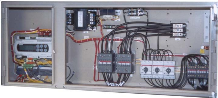
Figure 4, AGZ-A Control Panel
