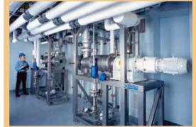
5 sq. ft. Artisan Rototherms® used for solvent recovery at a cGMP facility.
