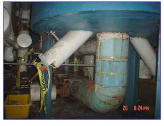
1994 Refrigeration Valves & Systems Corporation Ammonia Vertical Recirculator- 5 ft. dia. x 10 ft. 8 in. H. S/N: 94279. Nat'l Bd: 6718. MAWP: 250 psi @ 300°F. MDMT: -40°F @ 100 psi. Inlets: (1) 10 in. dia. port (suction in), (1) 2 in. dia. port (makeup liquid), (1) 3 in. dia. port (liquid feed). Outlets: (1) 8 in. dia. port (suction out), (2) 3/4 in. dia. ports (vents), (1) 6 in. dia. port (pump suction). Overall dimensions: 7 ft. 2 in. L x 6 ft. 6-1/2 in. W x 13 ft. 7-1/2 in. H.
