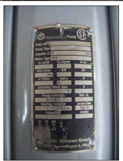
Hansen Technologies Hermetic Centrifugal Pump. Model: 2001. S/N: LCH93613. Type: CAM2/3. Maximum capacity: 52.7 gpm @ 105 tdh. Minimum capacity: 5.27 gpm @ 177 tdh. Impeller diameter: 4.48 in. Nominal pressure: 362 psi. AGX Motor, 4.56 hp (3.4 kW), 3400 rpm, 440 V, 7.5 amps, 60 Hz, 3 phase. Inlets: (1) 1-1/2 in. dia. flanged port. Outlets: (1) 1 in. dia. flanged port. Overall dimensions: 2 ft. L x 9 in. W x 10 in. H.
