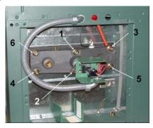
Fig. 8: Torque Sequence
