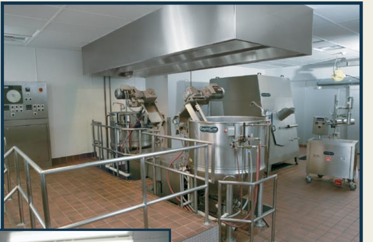
CapKold kitchen (from left to right, shown above) - kettle control panel, (2) kettles, tumble chiller and pump-fill station
