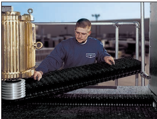
Water Saving Drift Eliminator
