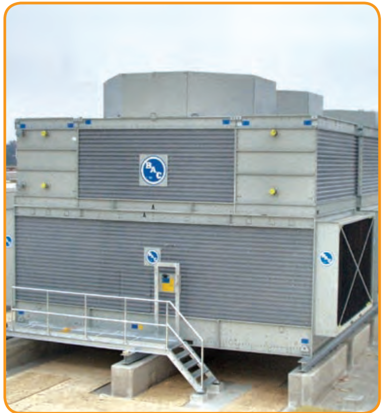
Unit with intake and discharge sound attenuation
