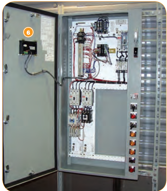
Enclosed Controls - (NEMA 3R Shown)
