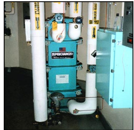
SUPERCHANGER heat exchangers recover heat very efficiently because of their high heat transfer rates and close temperature approach capabilities.
