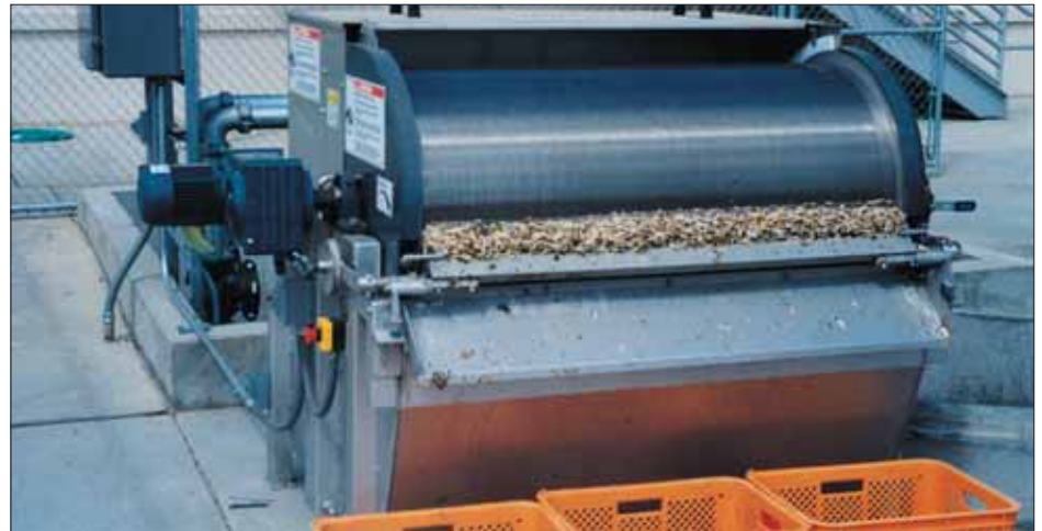
The Rotostrainer screens discrete solids, scum and oily materials without blinding
