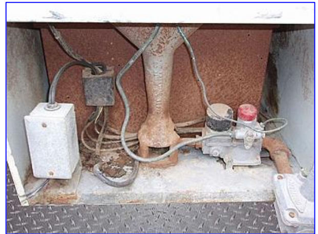
(3) L.B. White Direct Fired Circulating Construction Heaters. Model: 379G-1. S/N's: 19044. Capacity (input): 115,000 Btuh. Natural gas. Airflow: 480 cfm. Gas supply (max/min): 14/5.5 in. W.C. Burner manifold pressure: 4.5 in. W.C. Power supply: 115 VAC, 3 amps, 60 Hz, single phase. Overall dimensions: 23 in. L x 16 in. W x 24 in. H.
