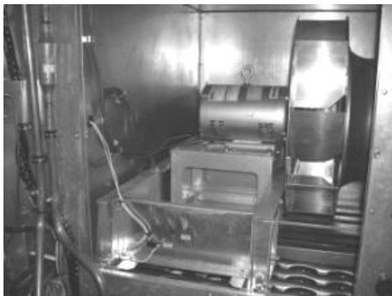
Figure 41 - 9-25 and 30 ton Supply Fan
