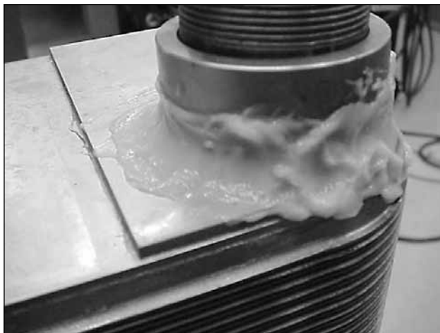
Figure 5 - Application of heat-sink paste before welding
